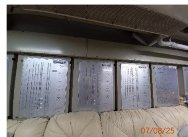
Graphic Annunciator Fire Alarm System
