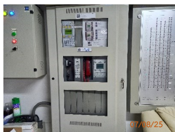
Fire Alarm Control Panel
